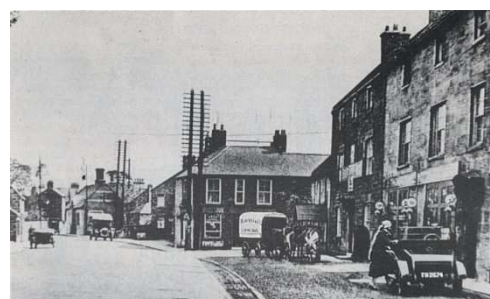
26. – ‘Ponteland’ (Main St. c.1930) In this photograph, provisions are still being delivered to the Seven Stars by horse-drawn van; the offices of the Ponteland Motor Car Co., are located in part of the former Albion Temperance Hotel; and Miss Kirkup, the chemist who occupied the rest of the ground floor, gets into her open-topped Morris.
