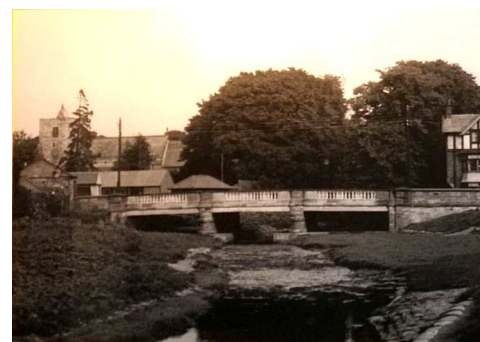
20. – Untitled (Ponteland Bridge c.1926) This postcard shows the widened bridge which replaced the old bridge in 1925. As well as removing a bottleneck on one of the routes to Scotland, it may have been hoped that the triple-span structure would provide easier flow and so reduce the chances of the river flooding.
