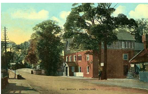
16. – ‘Bridge End & Smithy, Ponteland’. A nicely hand-tinted postcard subsequently re-issued as: ‘The Smithy, Ponteland’ shown here. Since the Diamond Inn has all the 2 nd -floor gables completed, the picture must date from about 1910 but before the old bridge was replaced by the present one in 1925.
